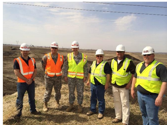
Charlie, Kenny and Larry with Corp of Engineers staff on the Consolidated North County Breach and Gravity Drain Project.
